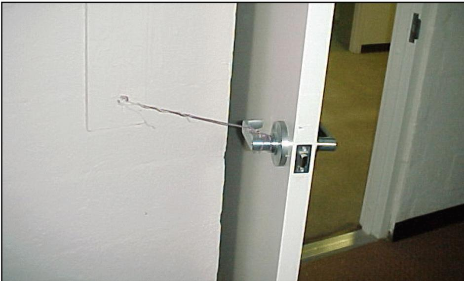
Figure 1: Fire door improperly held open by tying it to a wall.
