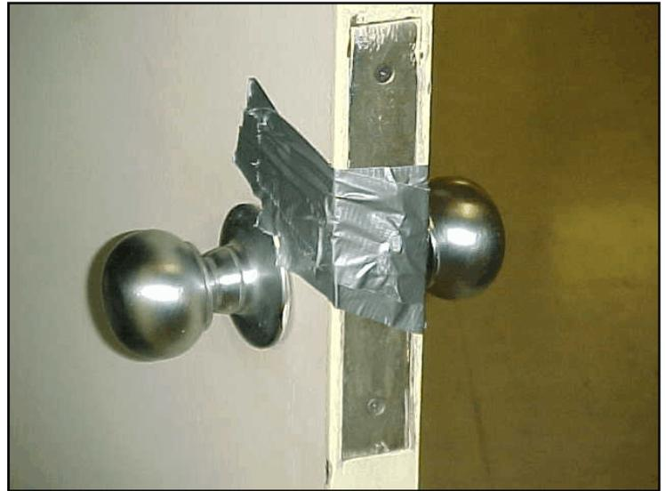
Figure 3: Fire door latch improperly taped to hold the door open.
