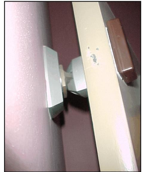
Figure 2: Electromagnetic hold-open device. This is the only means by which a fire door may be held open.
