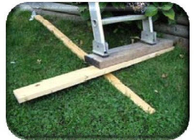
Improper footing
